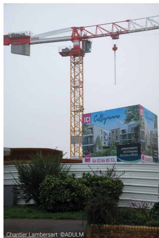
Chantier Lambersart ©ADULM
